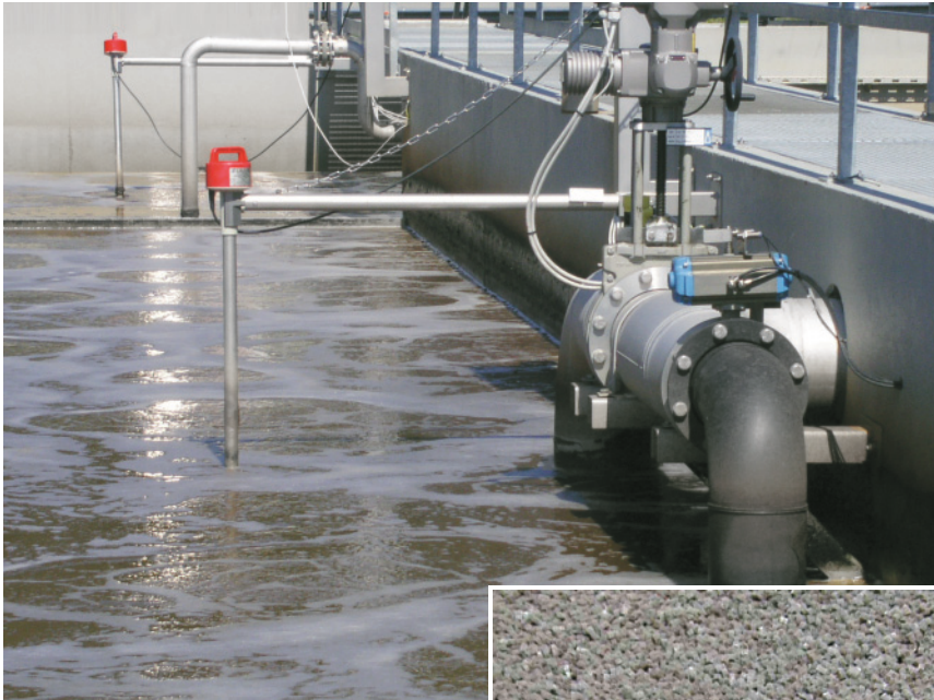
D.O. Probes in Sewage Treatment Application
