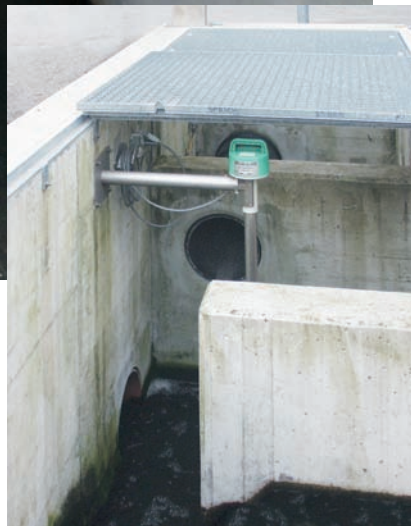
Inlet of a WWTP
